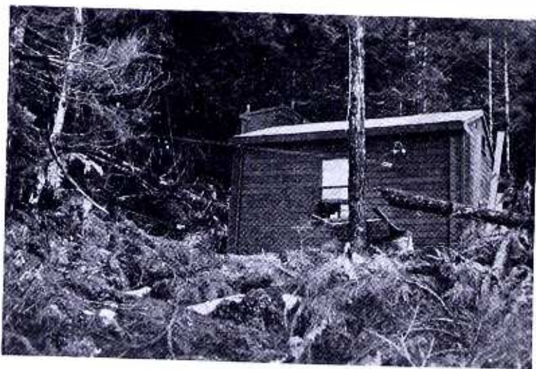
Fig. 24—Bella Coola Site. Pre-Fabricated Equipment Building.
