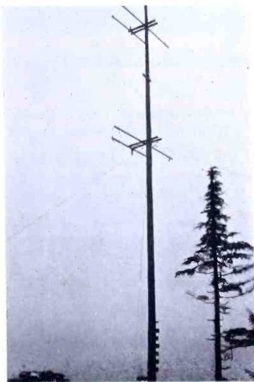
Fig. 22—Four-Element Antenna Array.
